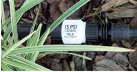
PRLG (Pressure Regulator Landscape Grade) is ideal for installations requiring lower flows of 0.5 to 7.0 gpm (114 to 1590 L/hr).
